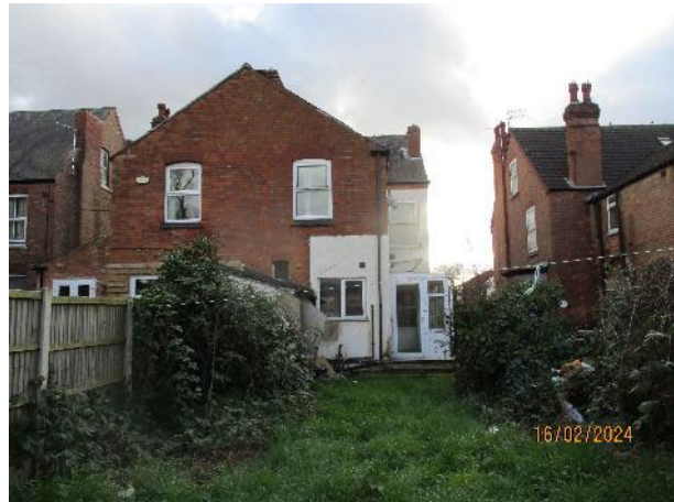
View of rear elevations
