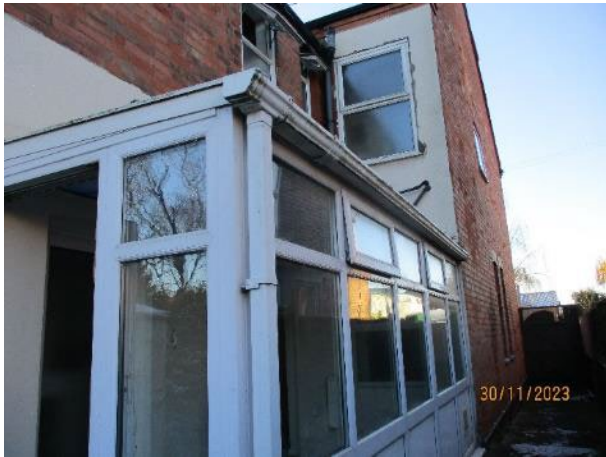
View of side elevations
